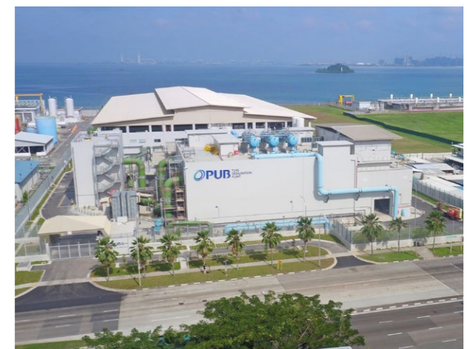
The Tuas Desalination Plant is the first in Singapore to be fitted with solar panels, with more than half of the total roof area covered by solar panels. The 1.2 MWp solar PV system will meet all of the energy needs of the plant's administrative building.
