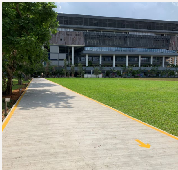
The 105m long footpath opposite Our Tampines Hub, which links to the Darul Ghufuran Mosque, is made from concrete which incorporates slag from processing municipal solid waste.
