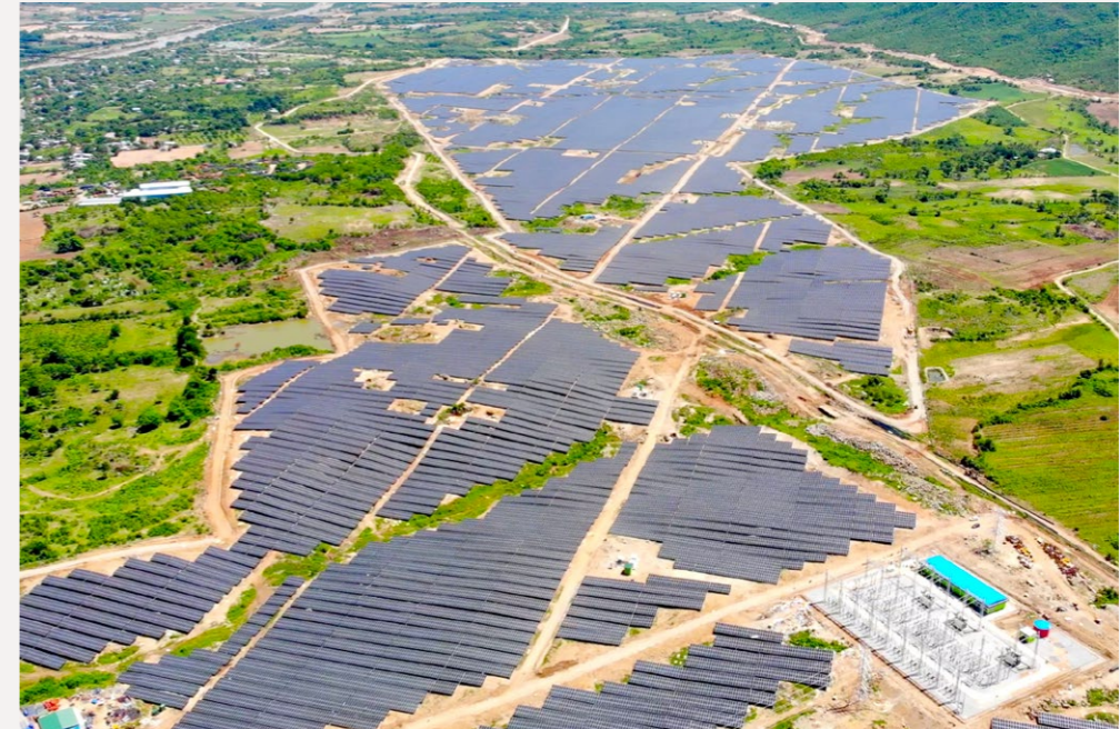
Sunseap's 168 MWp solar farm in Ninh Thuan, Vietnam is one of the largest in the country. Sunseap and InfraCo Asia contributed three billion Vietnamese dong (S$173,749) to fund the construction of concrete roads surrounding the site. At peak construction period, the project created over 2,000 jobs, mostly for locals in the area.
