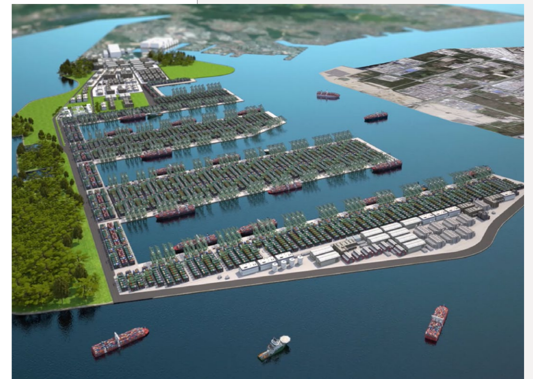
In addition to an automated wharf and yard that will raise efficiency, the waters around Tuas Port will be managed with a next-generation vessel traffic management system for safe and efficient navigation.
