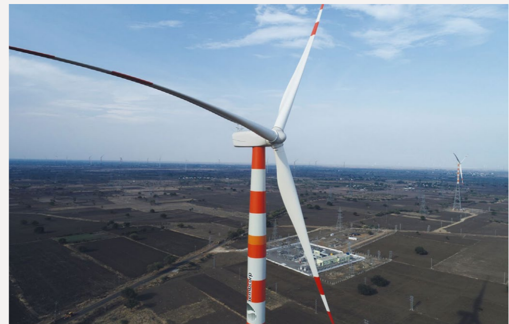
Sembcorp's 250 MW wind energy project in Tamil Nadu is the first reverse auction wind power project in India.
