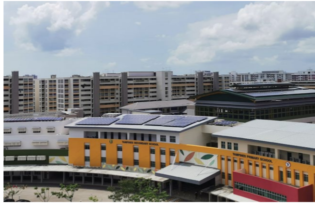
Tampines Secondary School is Singapore's first positive energy school with several innovative energy-saving solutions such as vertical greenery, enhanced sunshades, smart fans and solar panels.
