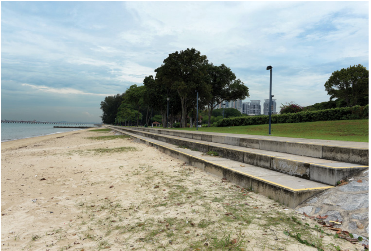
Composite stepped seawall at East Coast Park
