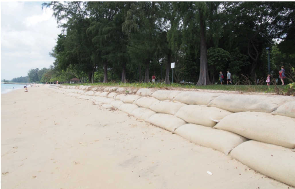
Geo-bags at East Coast Park
