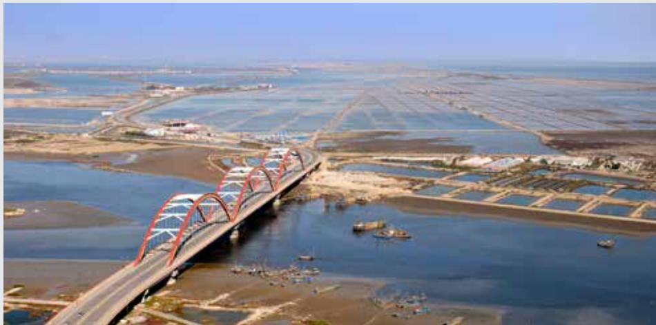
Bird's-eye view of the SSTEC in 2008. The original site comprised non-arable saline land and polluted water bodies.
