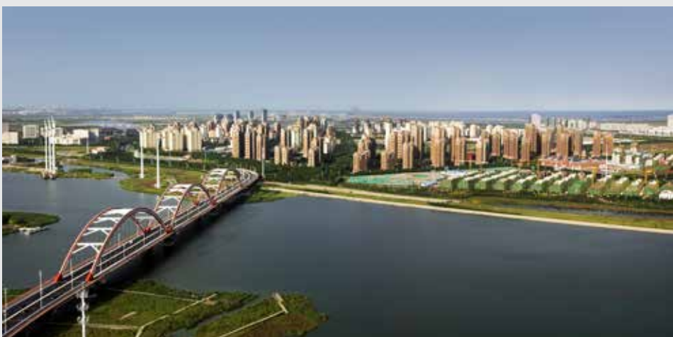
Bird's-eye view of the SSTEC in 2014. The site has since been transformed into a green city with tree-lined roads and lush landscaped housing estates.
