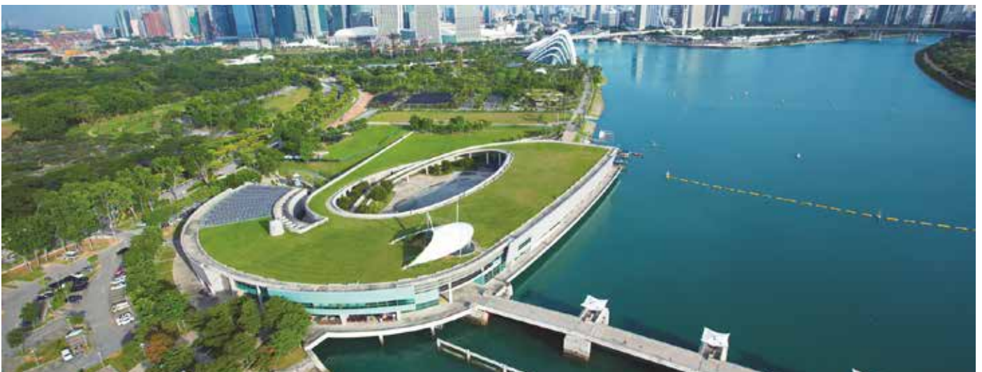
More than just an ordinary dam, the Marina Barrage serves three benefits: it creates a freshwater reservoir to boost Singapore's water supply, acts as a tidal barrier to prevent flooding in the low-lying areas in the city and offers a venue for water-based recreation.
