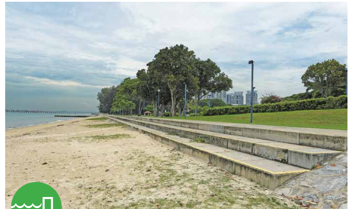
Composite stepped seawall at East Coast Park
