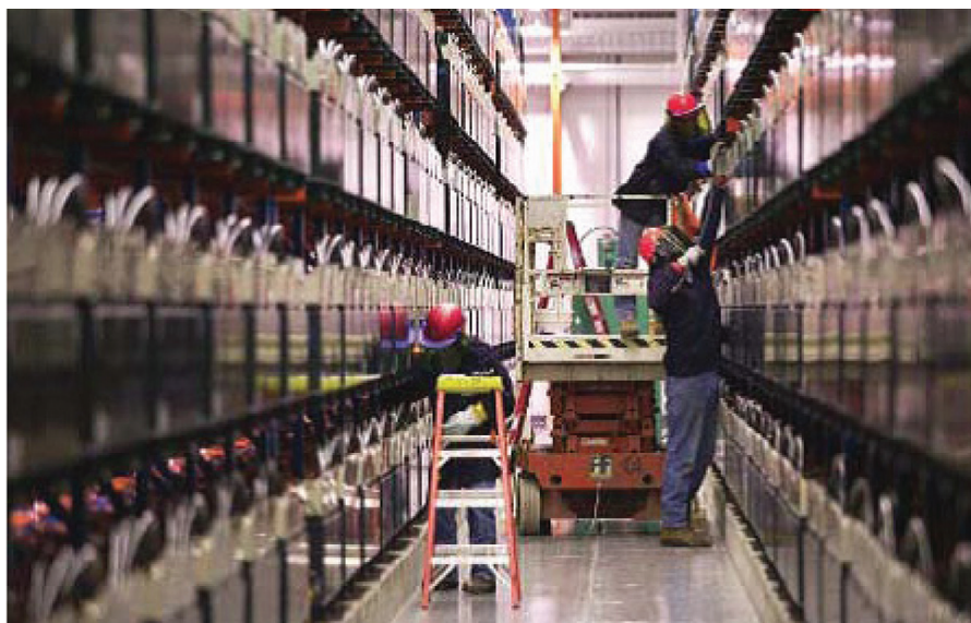
Figure A2: Golden Valley Electric Association (GVEA) located in Fairbanks, Ala, 13760 Saft SBH 920 high performance rechargeable nickel-cadmium cells 22
